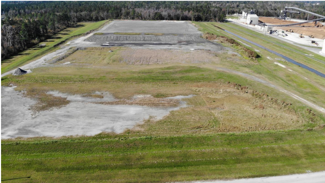
Figure 2. Aerial Image of CCR Landfill Facing West
